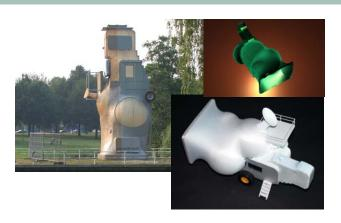
The design is achieved by means of an inflated membrane (inside) which supports the stressed shell (outside) This method is called the Blowing Structure Method. This methodology for the production of free form composite shells just obtained a patent
