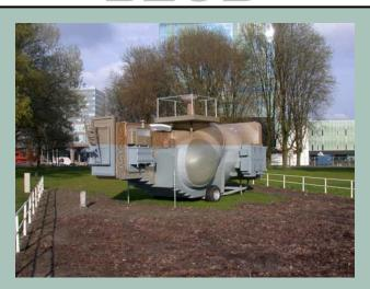
Here we see the concept and design for a artpavilion on the campus of the Technical University in Eindhoven. Its shell is made of glass-fibred polyester composite. The mould of the structure is made of PVC coated polyester membrane. The pavilion is used for exhibitions, films on a screen, as street lighting and as a piece of art. The pavilion can be used in 2 positions, vertically and horizontally.
