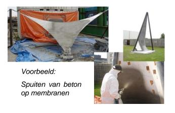
Modern innovative computer technologies make it possible to form double curved (freeform) architectural designs. Pneumatic and prestressed membranes / structures in combination with rigid elements play a major role in the development of these forms. Moreover, in this way also concrete and ice can be used as shell material
