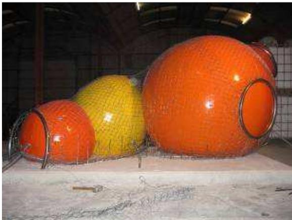
*Fig. 15 The balloons covered with wire mesh and the steel rings for the openings.*
