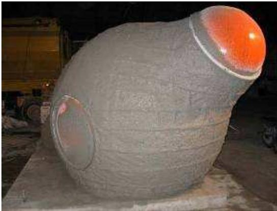
Fig. 16 Spraying the first layer of shotcrete .
