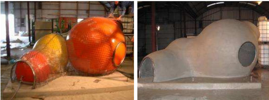
*Fig. 1, 2 Blob structure rigidised with shotcrete.*
